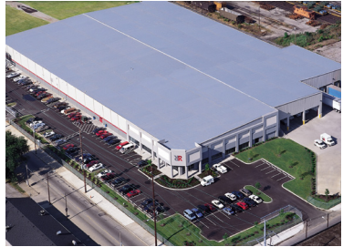
Shown is an aerial view of V.G. Reed & Sons' facility.
